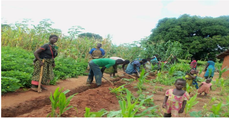
Men and women in trench digging for piped water distribution line in T/A Mwansambo in Nkhotakota
