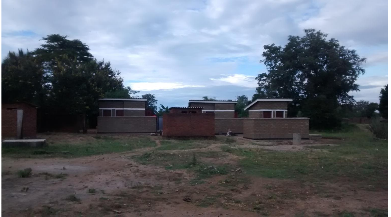
2 latrine blocks and 1 block wash room built at Mtosso Health Centre in Nkhotakota
