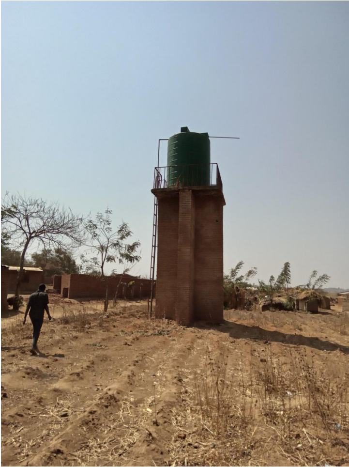
Reservoir and distribution tank that supplies water at Gumulira village
