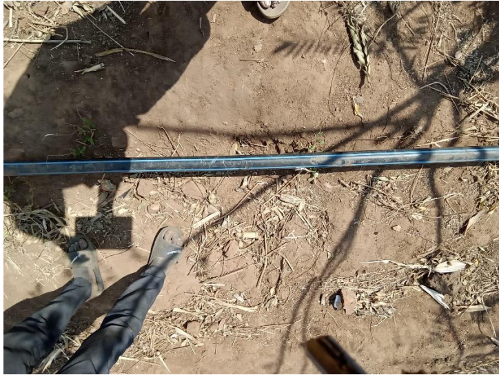
A section of 50mm pipe to be laid in a trench
