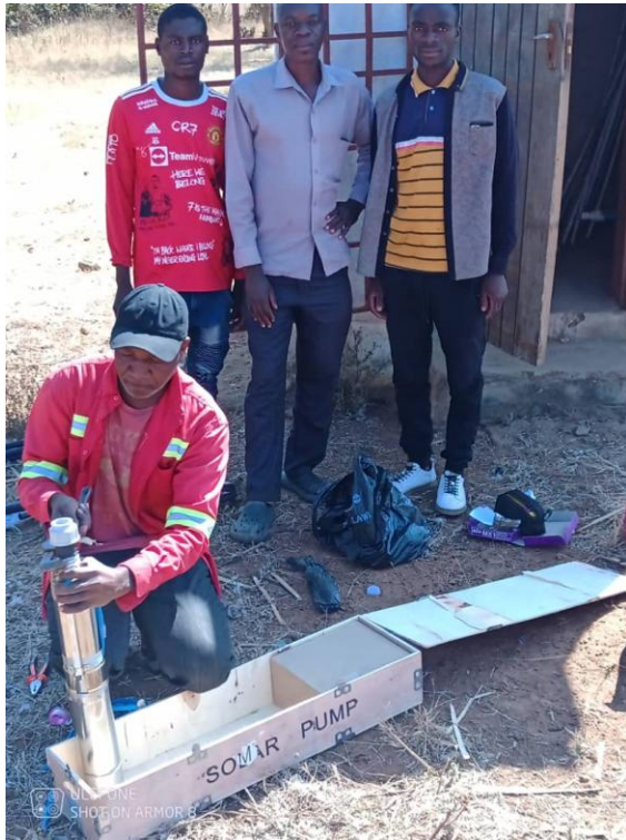
Unpacking the submersible pump prior to installation
